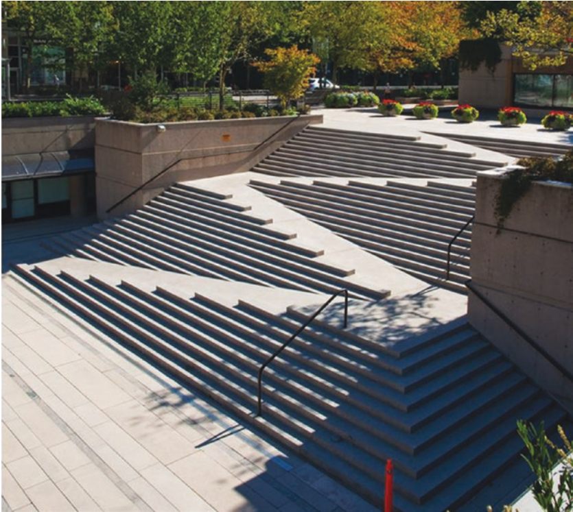
Figure 2-1. Photo of stairs with a ramp. Handrails are only on the stairs
